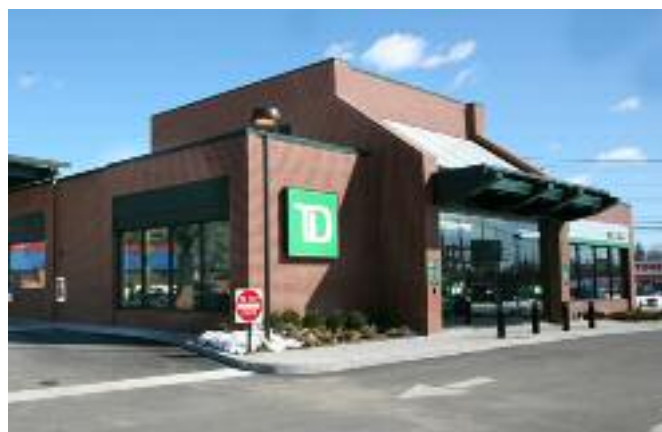
This branch in Farmingdale, NY, will be certified LEED gold in 2010 as part of our extensive LEED development program.
