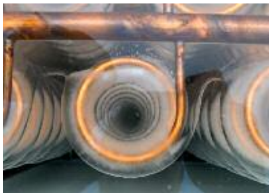
Ice Bear technology in London, Ontario: Large copper coils show how blocks of ice are frozen in tanks at night to cool the branch the next day.
