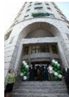
Unveiling of TD Bank sign at 1 Portland Square, Portland, MA
