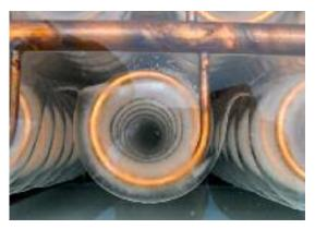
Ice Bear technology in London, Ontario: Large copper coils show how blocks of ice are frozen in tanks at night to cool the branch the next day.
